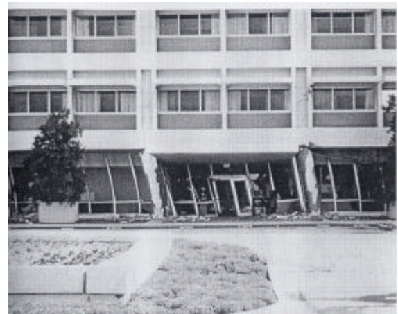
Soft story problem in San Francisco earthquake Olive view hospital, San Fernando earthquake
