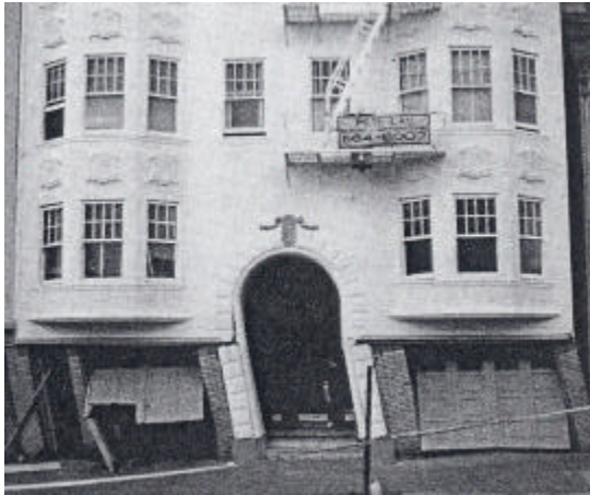
Soft story problem in San Francisco earthquake Olive view hospital, San Fernando earthquake
